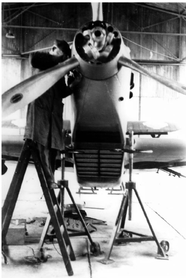
Georges Challess, Hispano Suiza technician works on HS 12Y29 engine installation in early 1938, at Zemun. Photo-Yugoslav Aviation Museum via Nenad Miklušev
